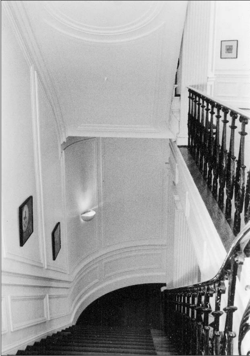
Staircase to Second Floor
